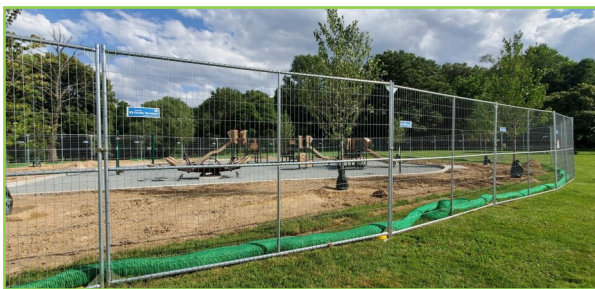
Fort Hunt Park’s new playground under construction
