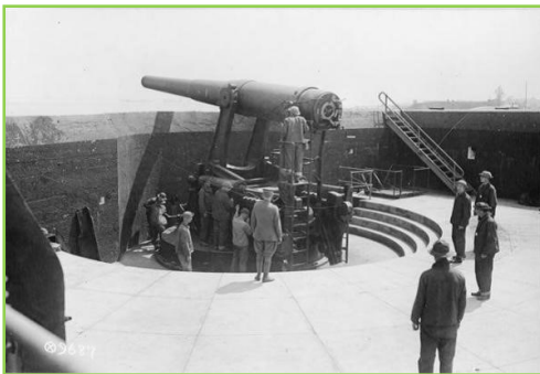
This 10-inch “disappearing gun” at Fort Monroe, Virginia, was similar to those on Battery Mount Vernon at what is now Fort Hunt Park. (picture from BikeWalkDrive.org)
